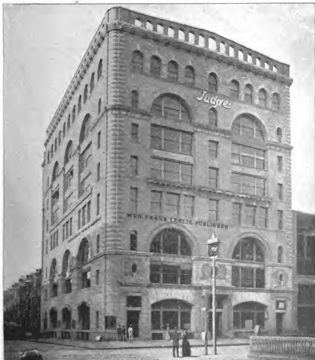
"JUDGE" BUILDING, THE HOME OF FRANK LESLIE'S PUBLICATIONS, FIFTH AVENUE AND 10TH STREET.
